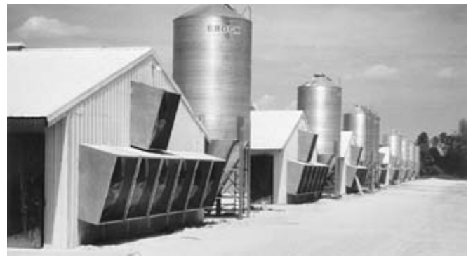
Fig. 1.2. Light-, temperature-, and ventilation-controlled houses exclude wild birds and most flying insects. Concrete aprons and paved roadways help prevent tracking of soil-borne diseases into the premises.
